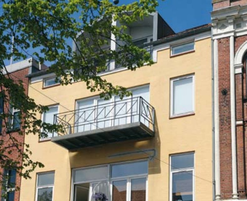
Indpasset facade, Kolding.
